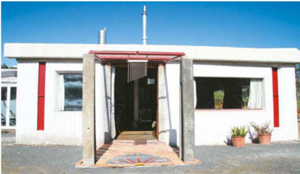
Above: Front entrance. The vertical red strips are louvres for ventilation. Photo: Sue Ferens
