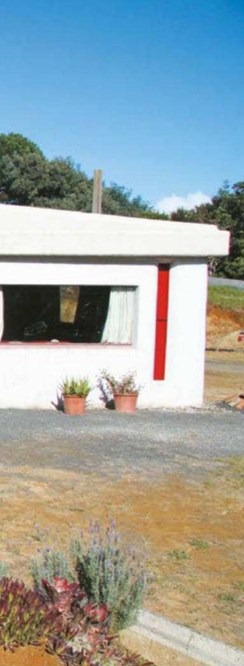
Above: This exterior view of Sean's house shows the simplicity of the two-room design. The conservatory forms the passage between the two wings and is also the bathroom. Behind the house is a prominent pole which holds the 1000-litre header tank. Photo: Sue Ferens
